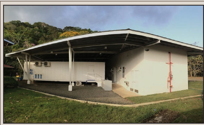
FIG. 2. The 5000 sq. ft. Gamboa Amphibian Research and Conservation Center has office space, telecommunications, laboratory space for visiting STRI researchers, a quarantine room, seven modified shipping containers, backup power, and waste-water treatment plant.
