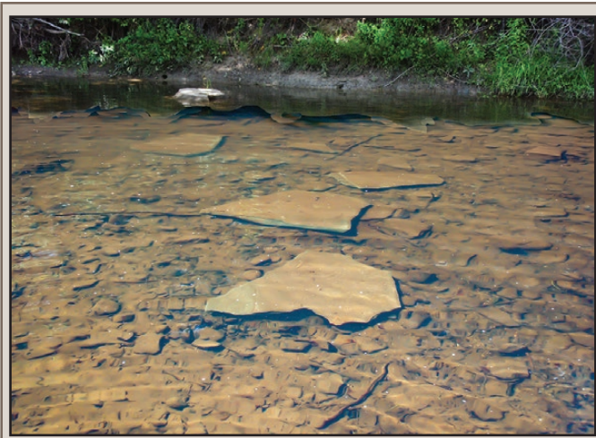
FIG. 2: Recently placed flagstone cover rocks.
